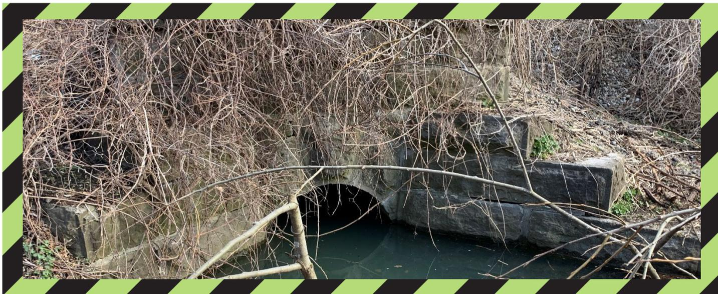
At the bottom of the Lakeshore East Rail Corridor embankment at Grey Abbey Park, water is unable to drain away causing water ponding and bank saturation. This is a serious safety issue for trains, their crew and passengers.
