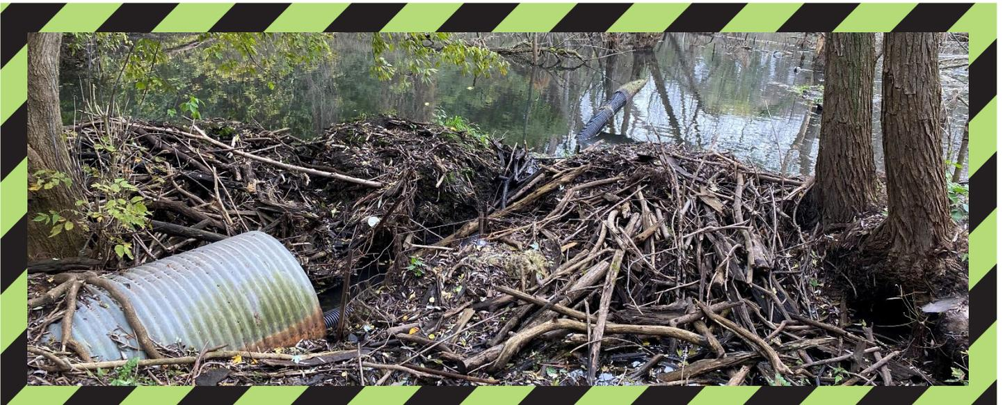
The culvert pipe is shown with the Beaver Baffle (corrugated plastic pipe) going through the beaver dam. The Beaver Baffle has been tampered with and pulled out of the water which prevents the water from flowing. This is a serious safety issue.
