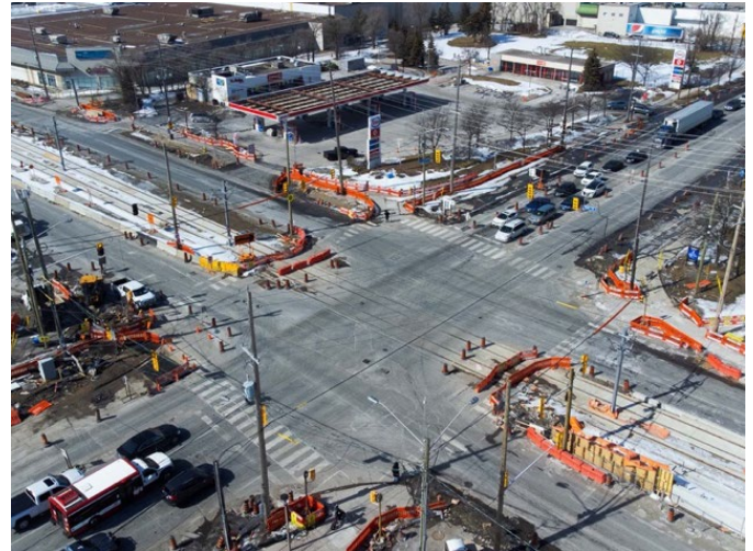
Photo: Intersection of Jane Street and Finch Avenue West.
