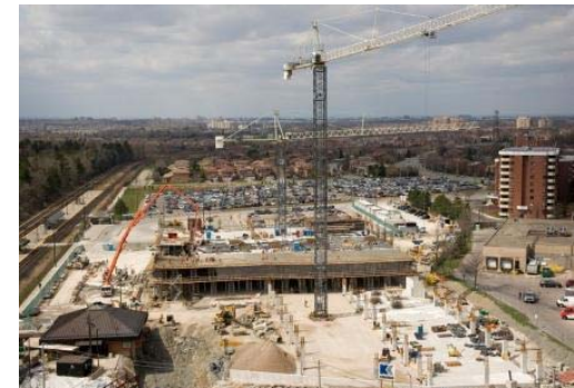
Construction of Erindale GO Parking Structure
