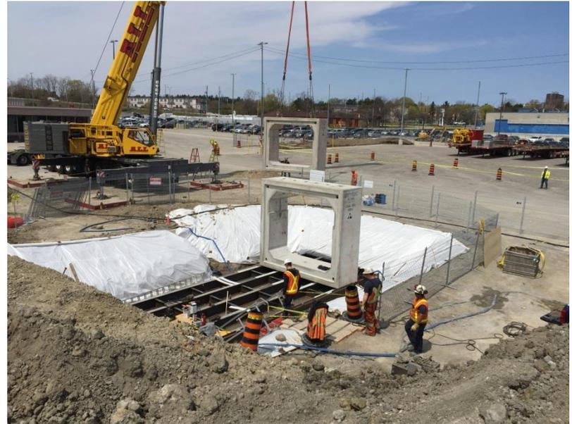
At Guildwood GO Station, the crane lifts precast tunnel sections and places on grillage in preparation for July tunnel slide work.
