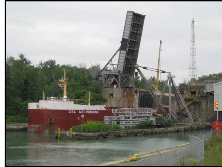
Figure 3.1 CNR “Bridge 6” Lift Bridge – Welland Canal
