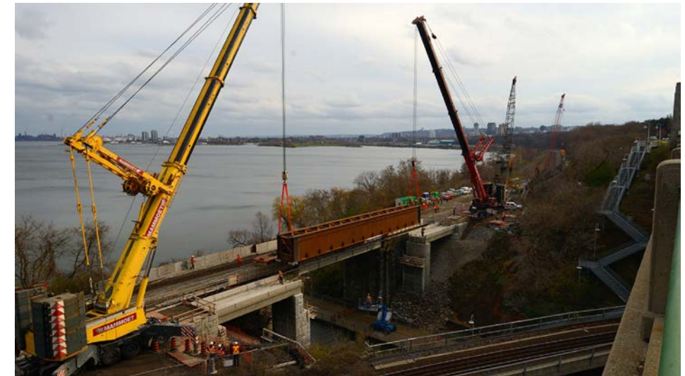
DESJARDINS CANAL BRIDGE EXPANSION
