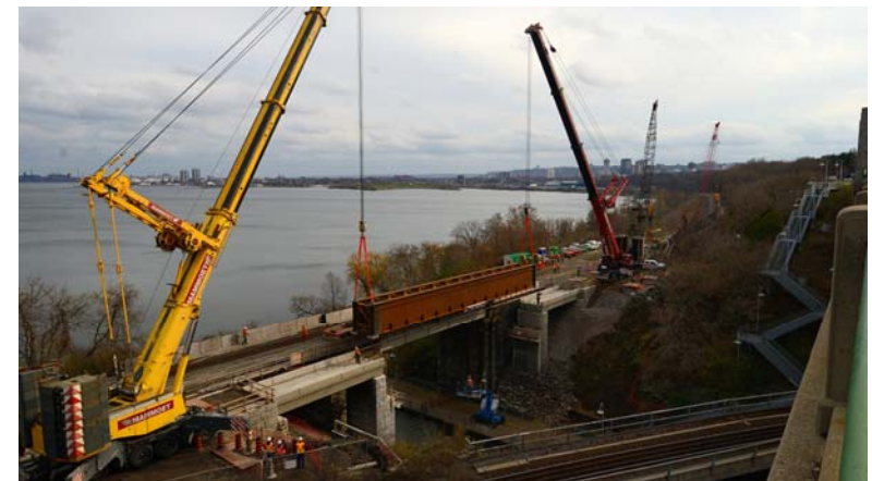
DESJARDINS CANAL BRIDGE EXPANSION
