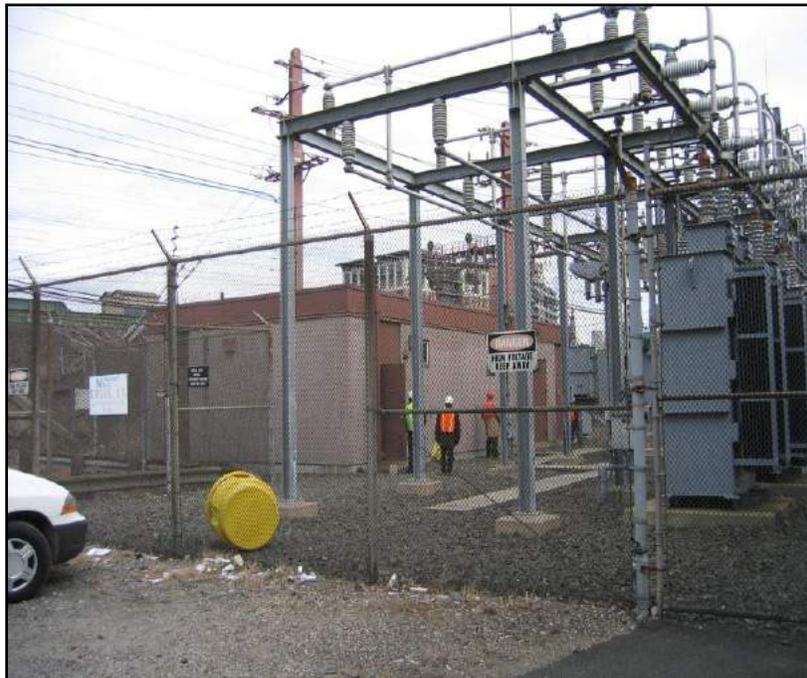
To ensure maximum reliability of the system, paralleling stations need to be located at regular intervals along the electrified route, approximately every 8 -12 km. There are two paralleling stations required as part of the electrified UP Express system: one at Ordnaunce Road, and one at 3500 Eglinton Avenue West (see **Figures 3-7** and **3-8** respectively). Further detail related to the process followed for identifying the preferred Paralleling Station locations is contained in Chapter 2.
