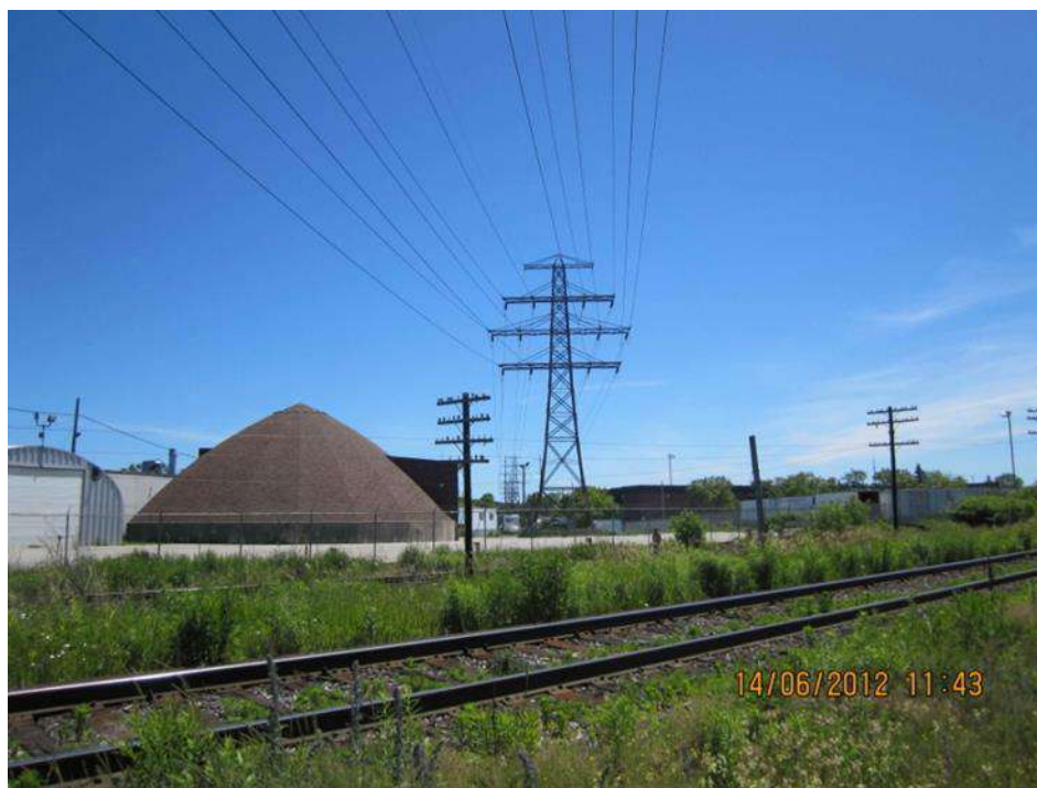
Figure 4-1 Mile 5.7 Weston Sub. - Overhead Transmission Lines
