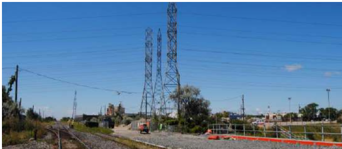
Figure 9-3 Hydro One Transmission Lines Crossing the Railway (Milepost 11.1)
