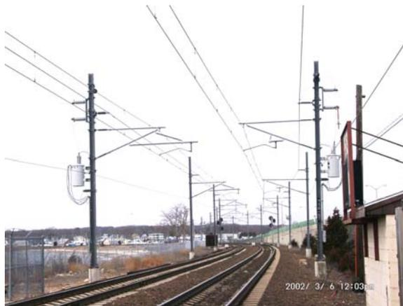
The OCS poles are installed at both sides of the track and are spaced approximately 55-60 m apart on tangent track, with the spacing decreasing progressively with decreasing radius of curves.
