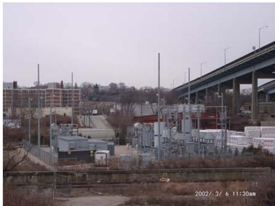
**Figure 10: Typical 2x25 KV System Autotransformer Station**
