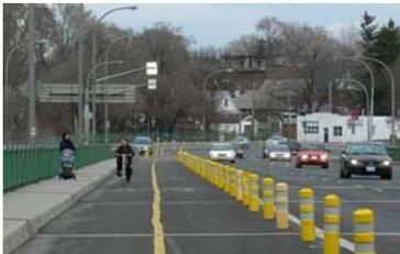
*In Hamilton, one lane of arterial traffic was converted to a two-way bike path, allowing cyclists to safely cross Highway 403*
