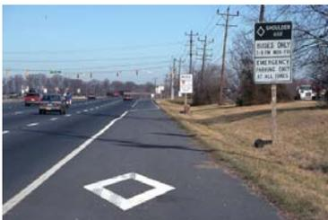
US 29 near Washington D.C. allows buses to bypass signal queues by operating on the paved shoulder
